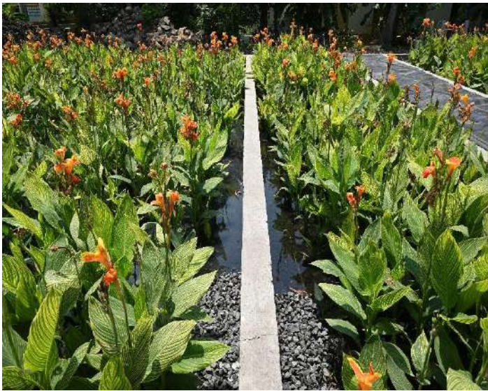
IWT – Green Sewage Treatment Plant Installed at Township
