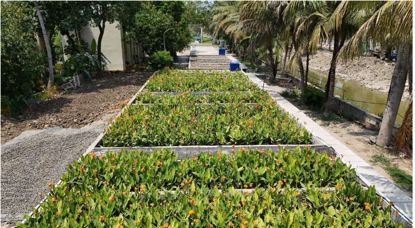
IWT – Green Sewage Treatment Plant Installed at Township
