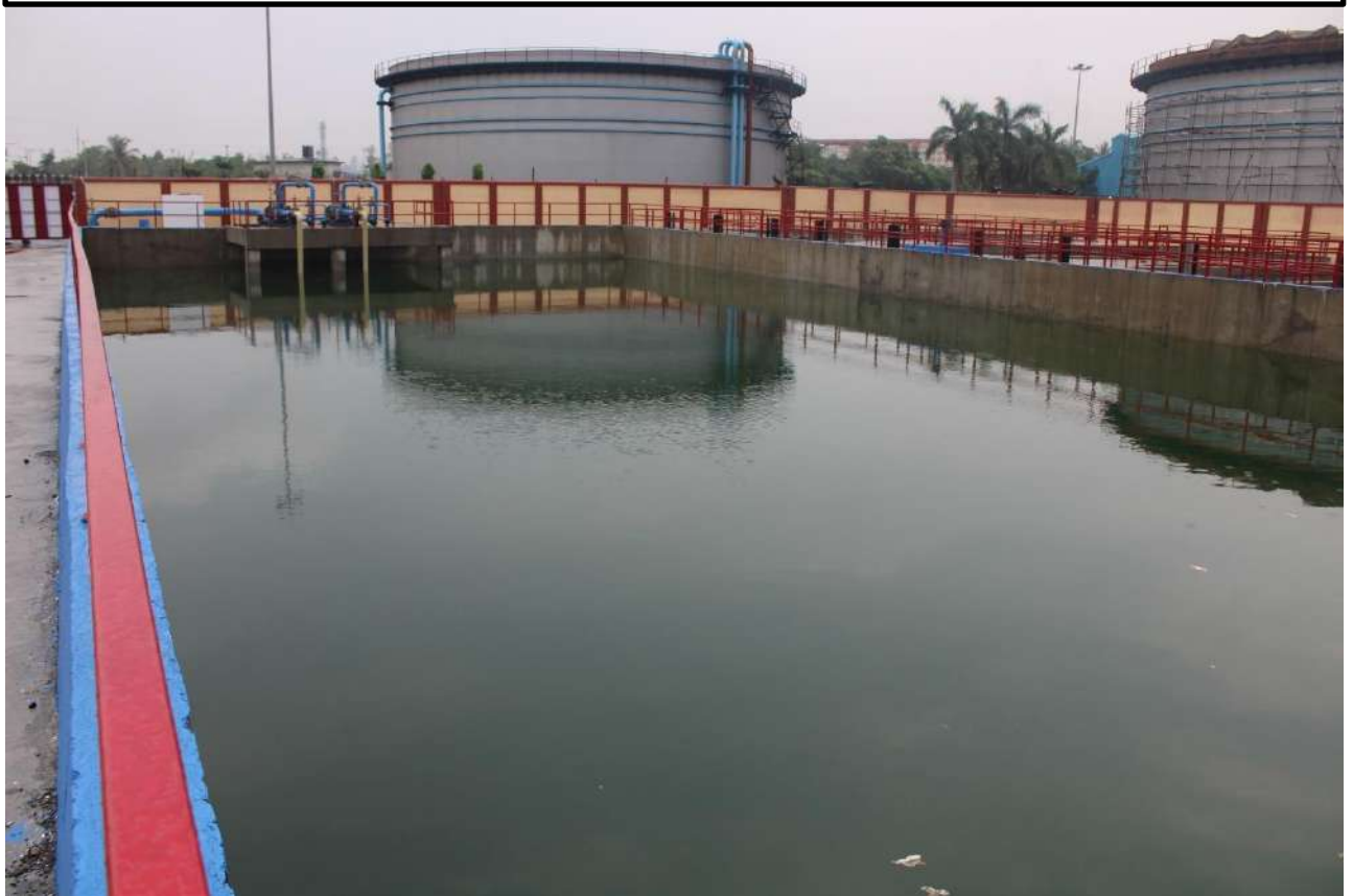
Neerkund - Constructed on a 46m x 23m footprint with an average depth of 6 meters, Neer Kund offers a net holding capacity of 3800 m 3 .
