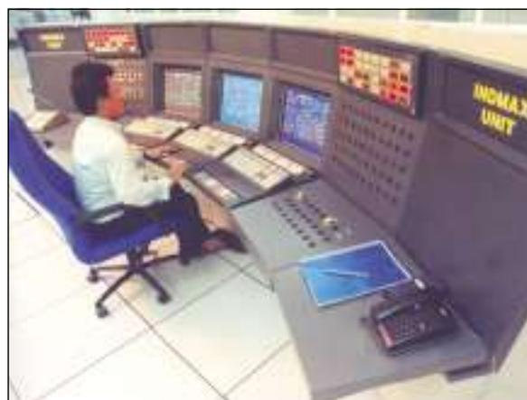
Control panel for IndMax unit at IndianOil's Guwahati Refinery - a proprietary technology for maximising LPG yield.
